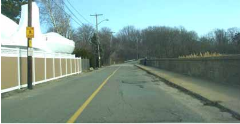
Looking east on Winter Island Drive near sea wall
