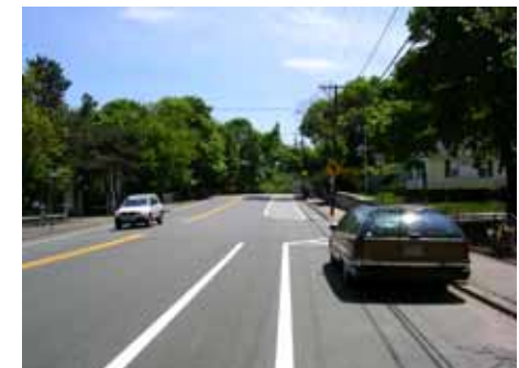
Looking south on Lafayette Street at Raymond Road to new bike lane markings
