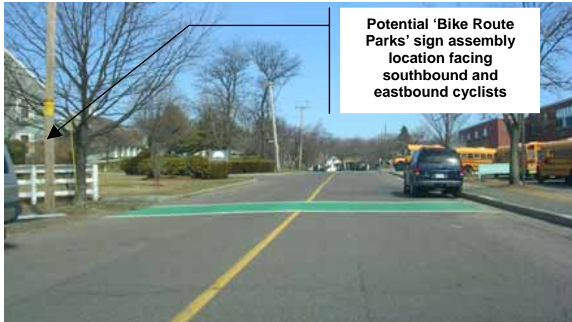
Looking north on Szetela Lane at Pilot Route crossing
