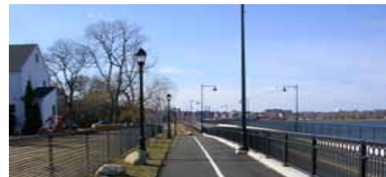
Looking south – Bypass Road Multiuse Path
