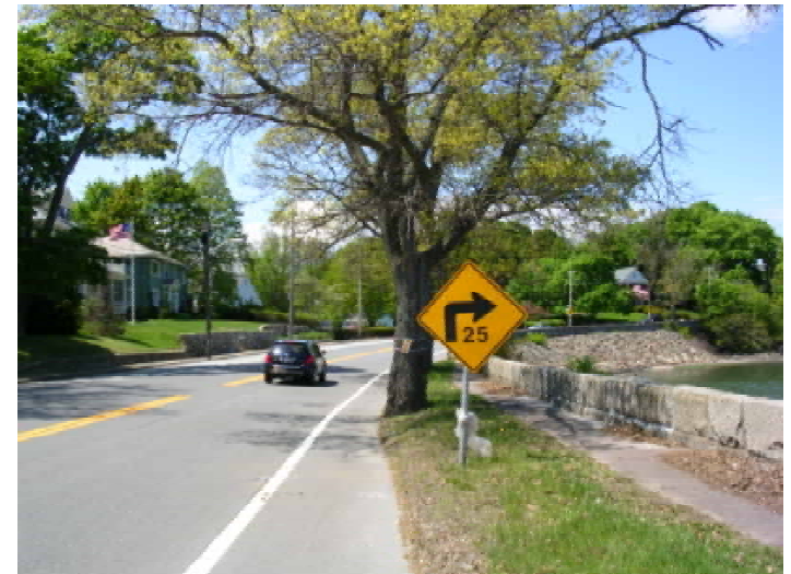
Lafayette Street looking to northbound Bike Shoulder
