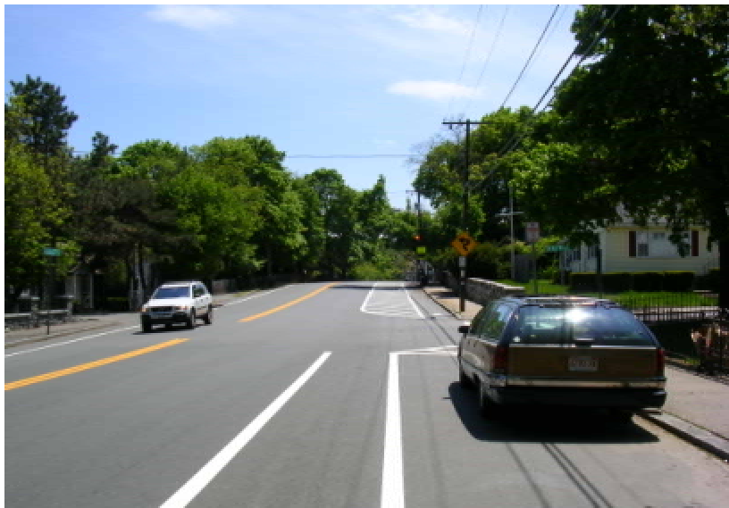
Lafayette Street looking southbound to Raymond Avenue at New Bike Lane
