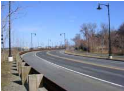
Looking northeast across Bridge Street from multifamily site
