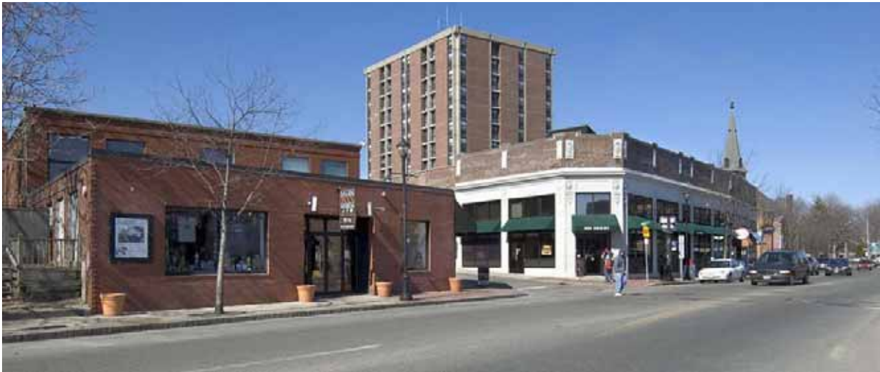
Lower Derby Street showing former industrial and automobile showroom buildings from the 1920s rehabilitated for retail uses.
