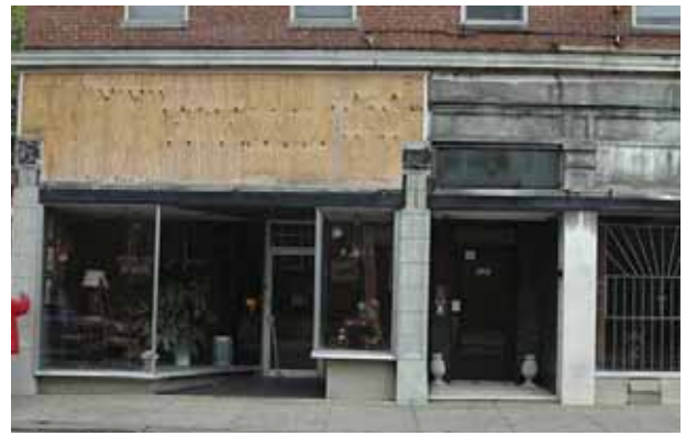
The historic sign band and transom windows seen at the right can be used to attempt an historic restoration of the missing façade at left.
