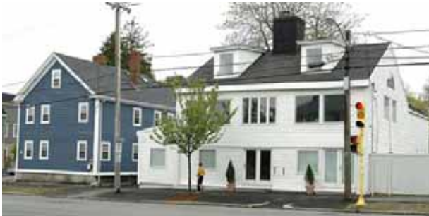
Eighteenth century house insensitively remodeled for commercial use with oversized modern windows. House at left retains traditional style windows.
