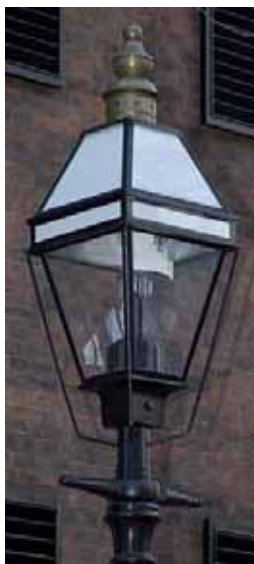
Recommended: A functional lighting fixture, as shown above, directs light downward onto the site. Historic fixtures, as shown on the left, should be used only with low wattage lamps to reduce glare.
