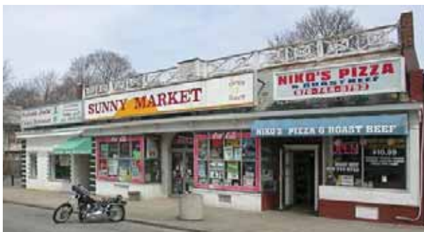
Retail block originally designed to fit into the neighborhood with an attractive balustrade and pitched slate roof now obscured by signage.
