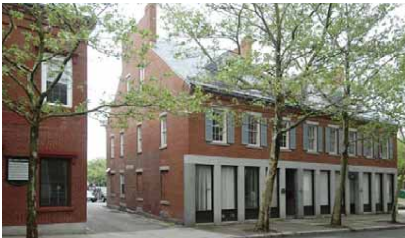
Current photograph of 17–23 Front Street shows the windows and dormers of the upper floors have been restored. The granite pier and lintel storefront system has been reconstructed following the evidence provided by the historic photograph. The glazing uses a modern system of insulated glass rather than restoring the small pane wood storefront windows visible in the historic photograph. In other similar buildings restored on Front Street, small pane windows were used to create a more accurate appearance.
