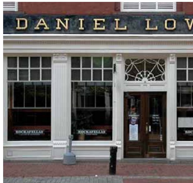
Salem's historic buildings have been transformed for new uses with sensitive rehabilitation that preserves significant historic elements such as this 1890's cast iron storefront.
