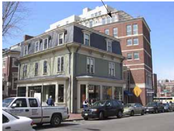
The upper two stories of this new building is stepped back away from the street and neighbors to reduce the visual impact of it height. (Cambridge)
