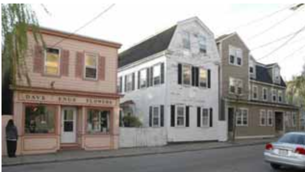
Derby Street east of the Custom House is characterized by a mixture of eighteenth and nineteenth century residential buildings and early twentieth century retail conversions.
