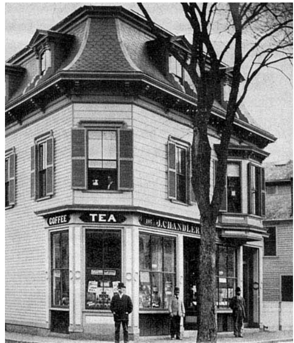
A similar wood storefront with more elaborately decorated piers and typical nineteenth century signs inserted in a Federal Street house. Courtesy of The Peabody Essex Museum.
