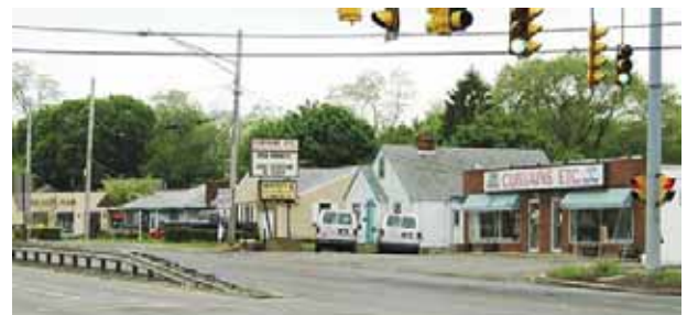
Older commercial construction along Highland Avenue often lacks well defined curb cuts and landscaped buffers, and it's sometimes interspersed with residential uses.
