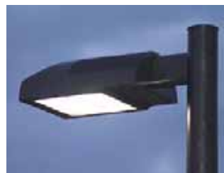
Recommended: A functional lighting fixture, as shown above, directs light downward onto the site. Historic fixtures, as shown on the left, should be used only with low wattage lamps to reduce glare.
