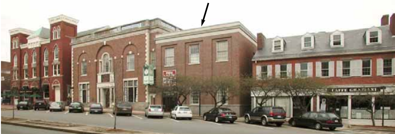
Current photograph of east side of Washington Street showing a rehabilitated late Federal Period building on right and a new infill building in center (marked with arrow). The cornice height of the new building has been sensitively located midway between the cornices of the flanking buildings. It uses brick with simplified traditional detailing in a manner that does not visually compete with the adjacent Colonial Revival bank building.
