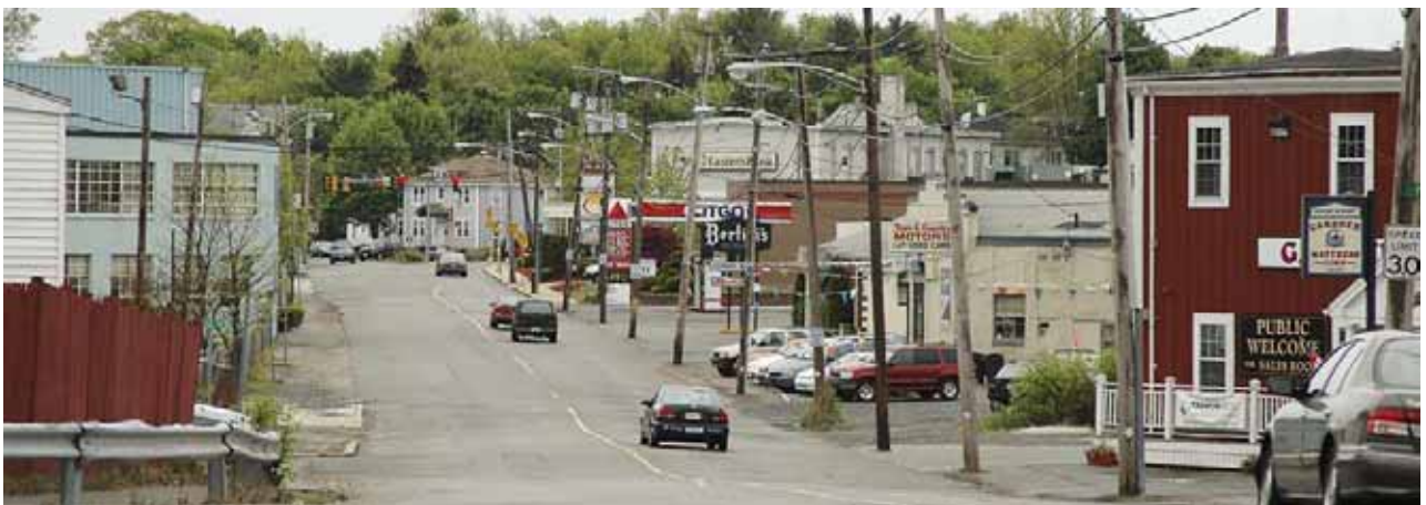
Western end of Canal Street looking south towards Loring Avenue showing chaotic mixture of commercial buildings, parking lots, and lack of sidewalks.
