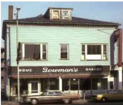
The 1761 Orne House on Essex Street in 1980 with its original architecture obscured by artificial siding and oversized windows. The ground floor was converted to retail use in the early twentieth century. The storefront in this picture dates to the 1950s. Courtesy of City of Salem.
