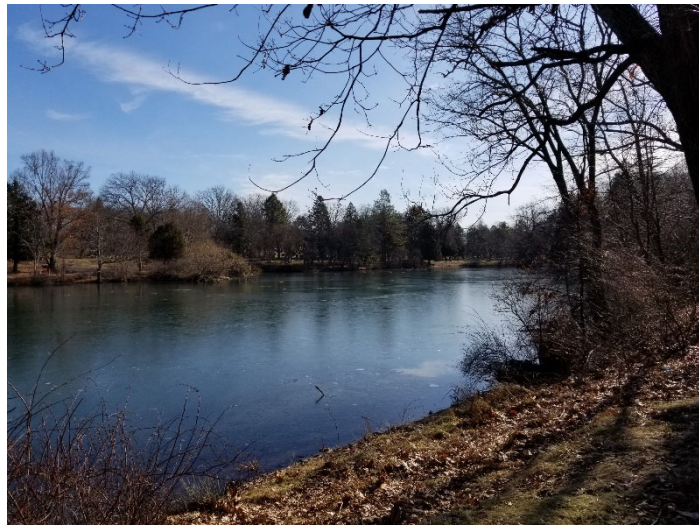
The condition of Greenlawn's ponds, including algae bloom, edge erosion and stagnation of water, emerged as an area of major concern to the public.
