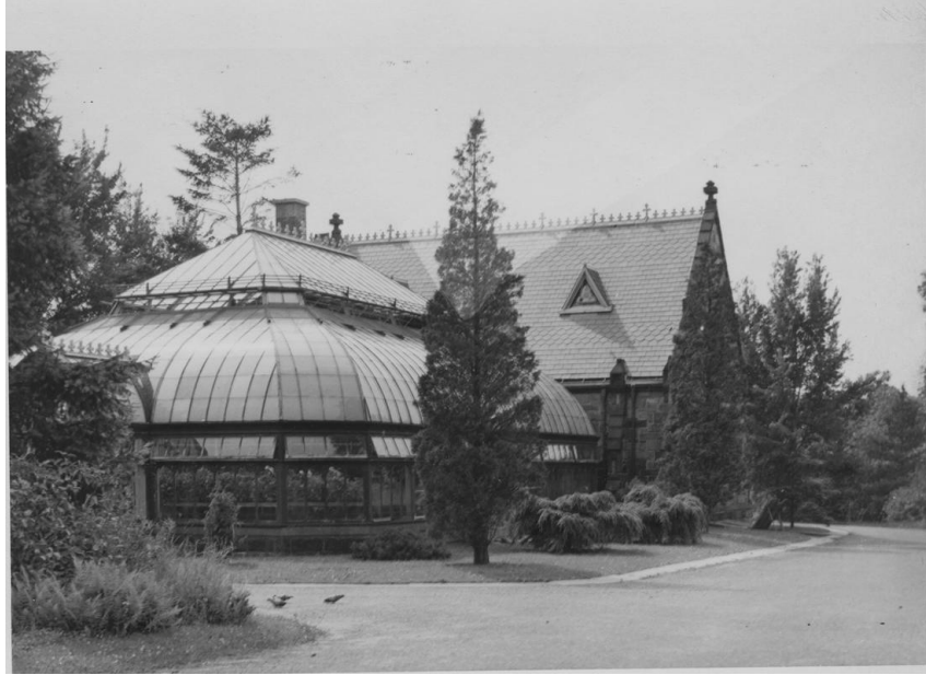
The conservatory attached to the Dickson Chapel contained a two-tiered glass roof which remained until it was removed in 1982. The foundation remains. (Collection of the Phillips Library, Peabody Essex Museum)
