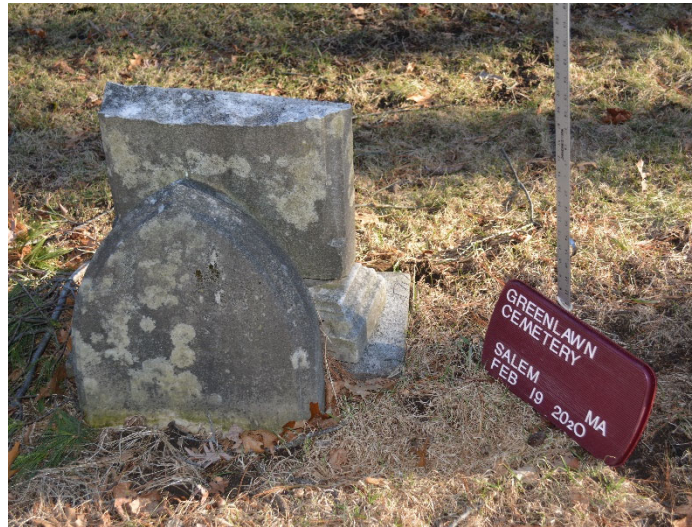
Many of the gravestones in the "Old Section" exhibit multiple types of deterioration, including breaks in the stone and build up of biological growth on the stone surfaces.
