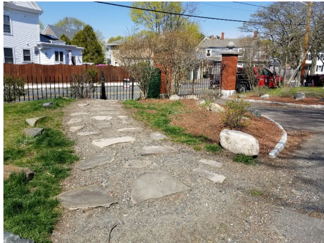
An informal pedestrian gate stands alongside the Liberty Hill Gate. Its gravel and stepping stone pathway leading into the cemetery does not meet ADA guidelines.
