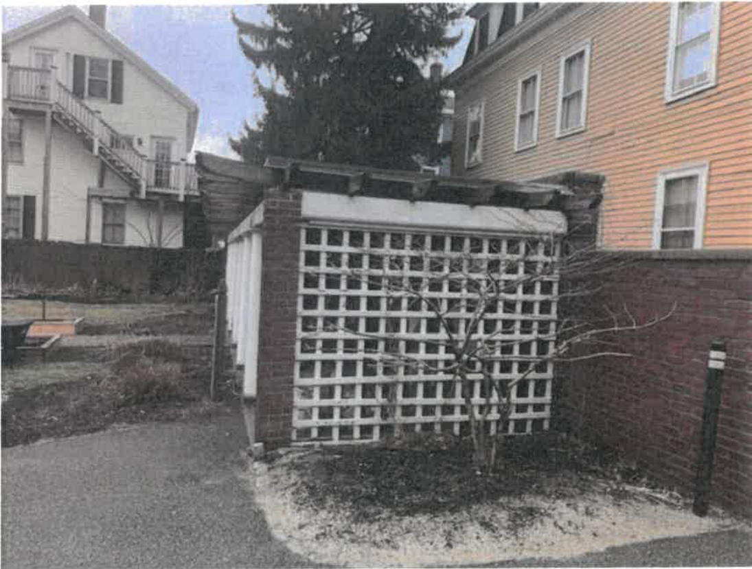
Photo #18 – View of open air shelter East facade
