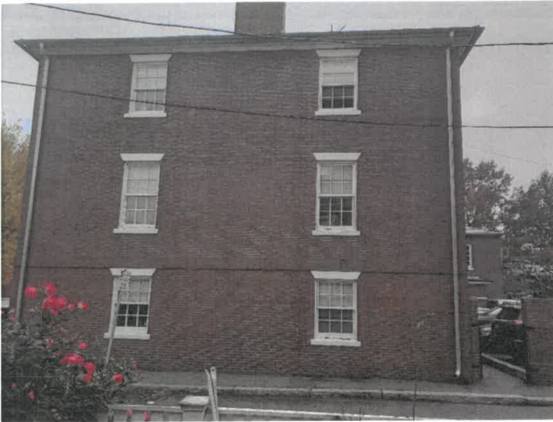
Photo #7 – View of rear façade (North), Curtis Street
