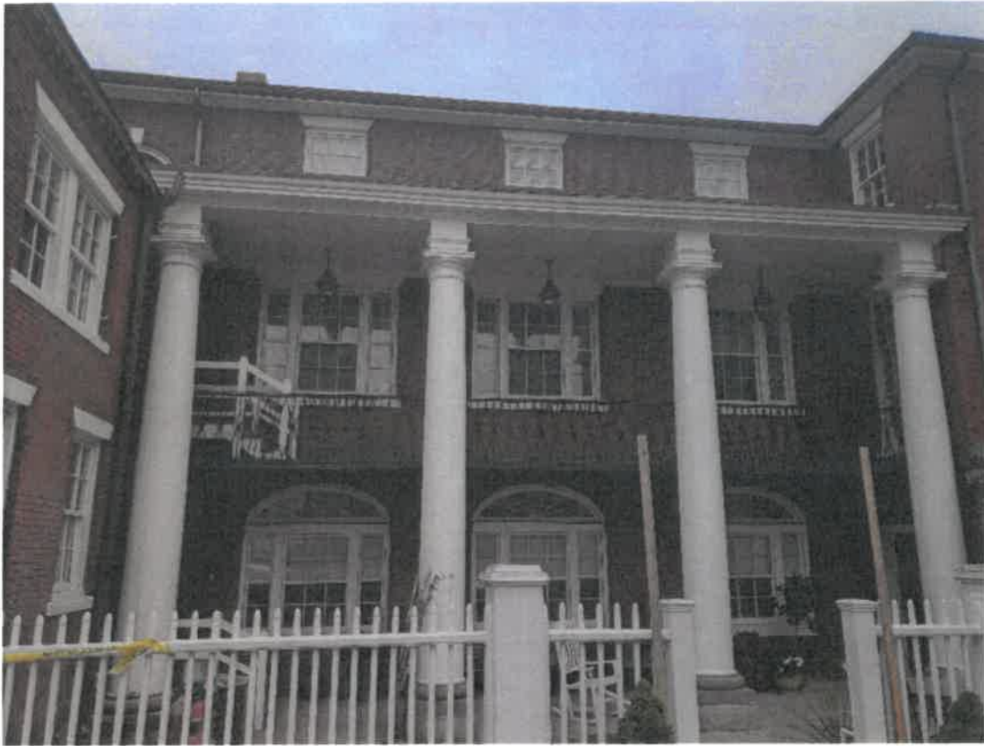
Photo #13 – View of West façade from interior of lot, courtyard
