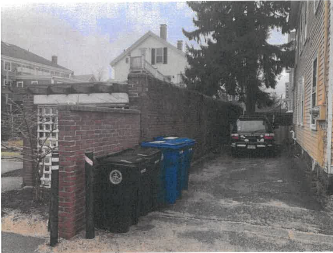
Photo #19 – View of rear wall of popen air shelter North façade
