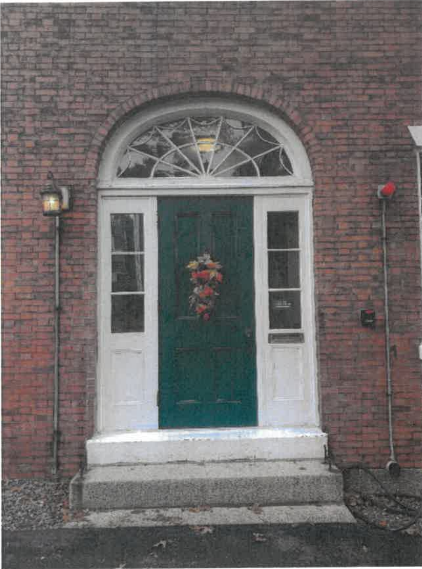
Photo #16 – Detail of West façade entrance
