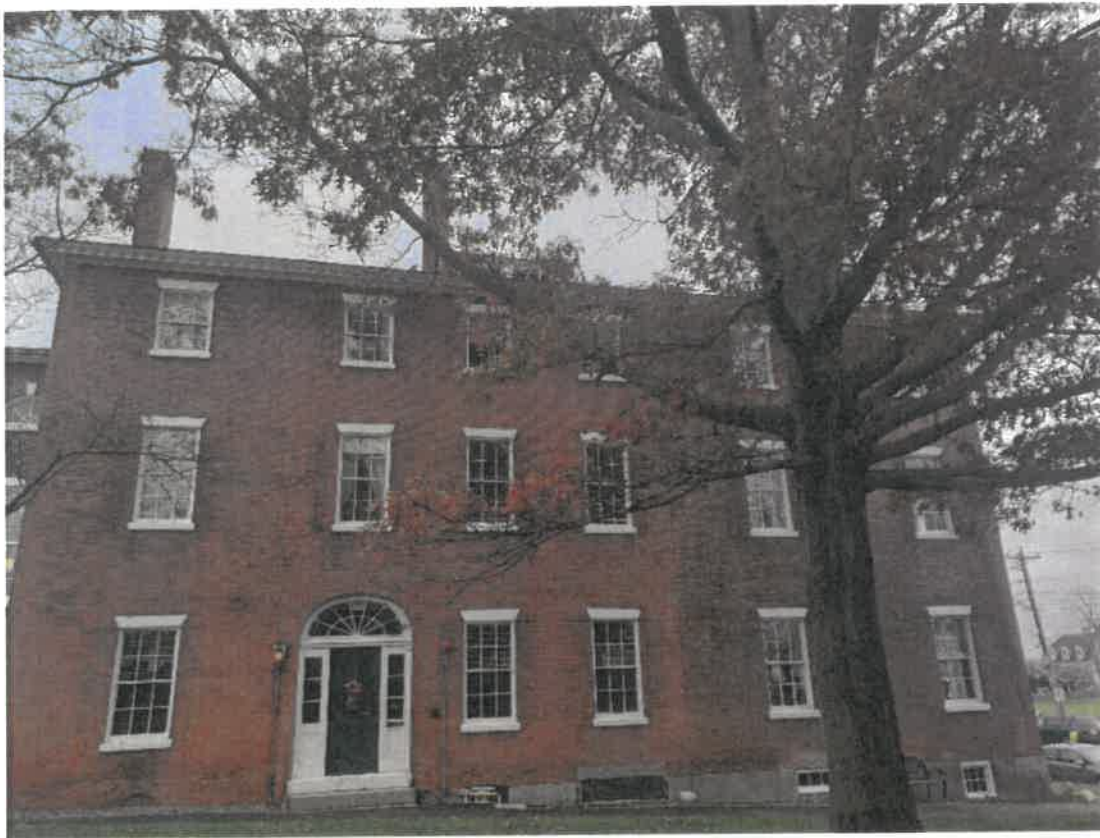
Photo #15 – View of West façade from interior of lot, front section
