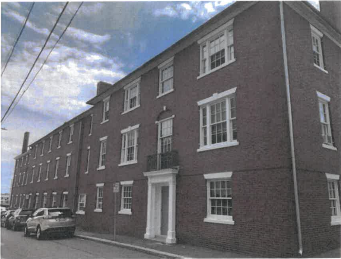
Photo #5: Orange Street façade (East) – view of rear section from corner of Orange & Curtis Streets
