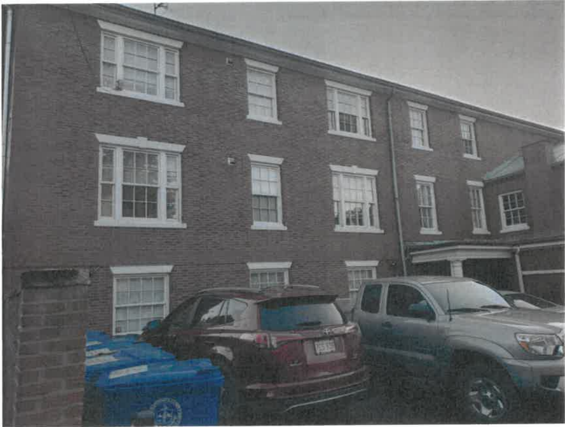
Photo #9 – View of West Façade rear section from Curtis Street
