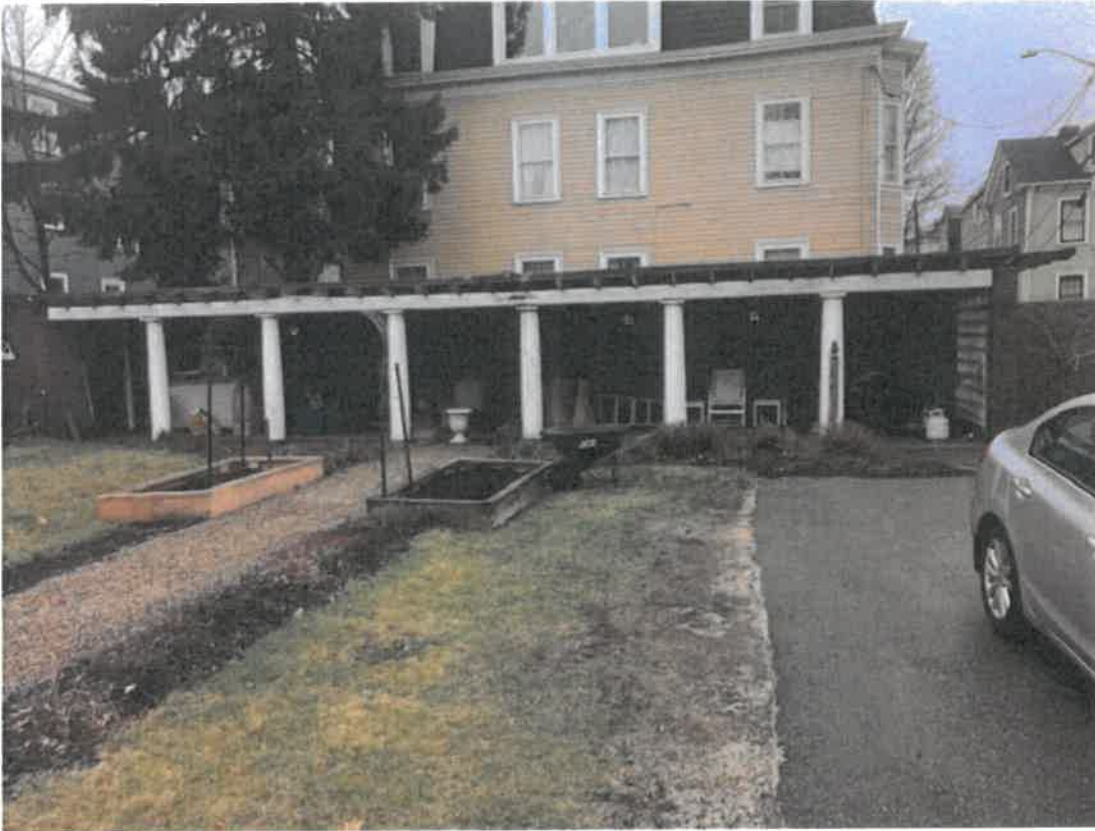
Photo #17 – View of open air shelter South facade
