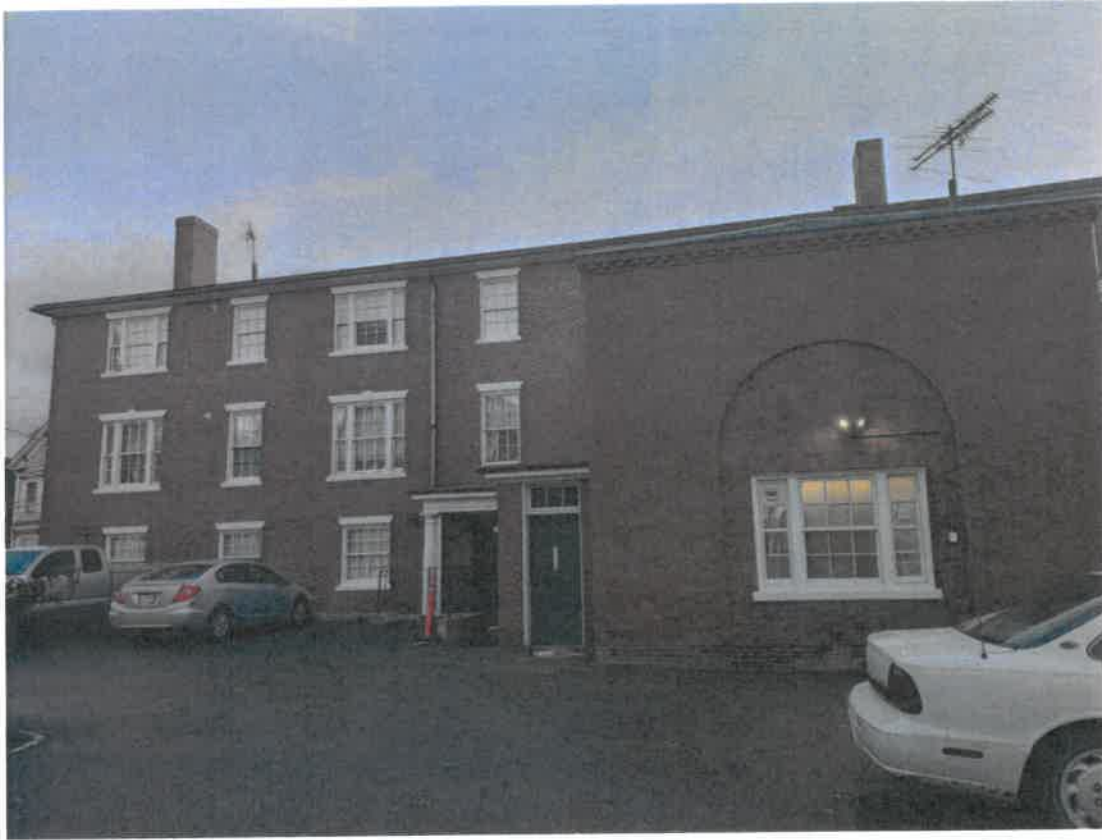
Photo #11 – View of West Façade from interior of lot, rear section
