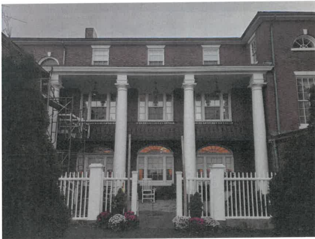
Photo #12 – View of West façade from interior of lot, courtyard
