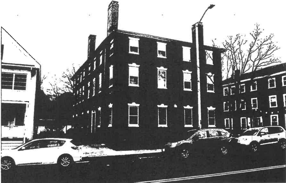
1. Main Block - South and East Elevations
