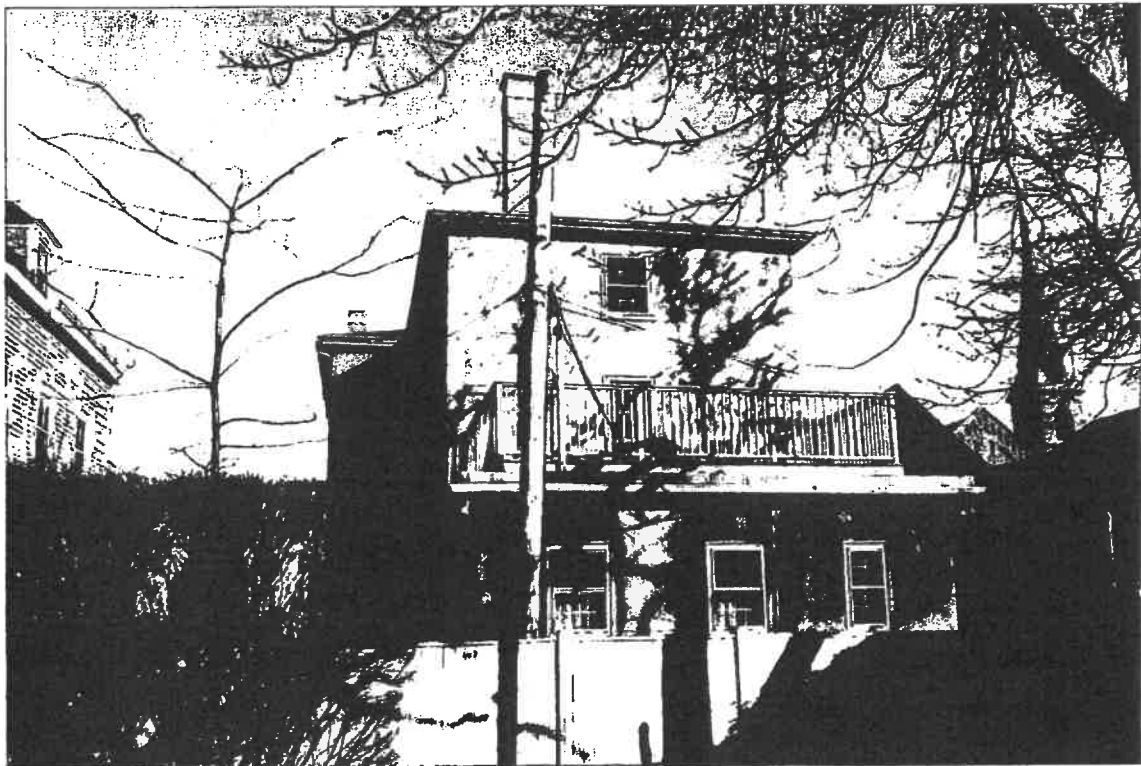
10. Ells - West Elevations
