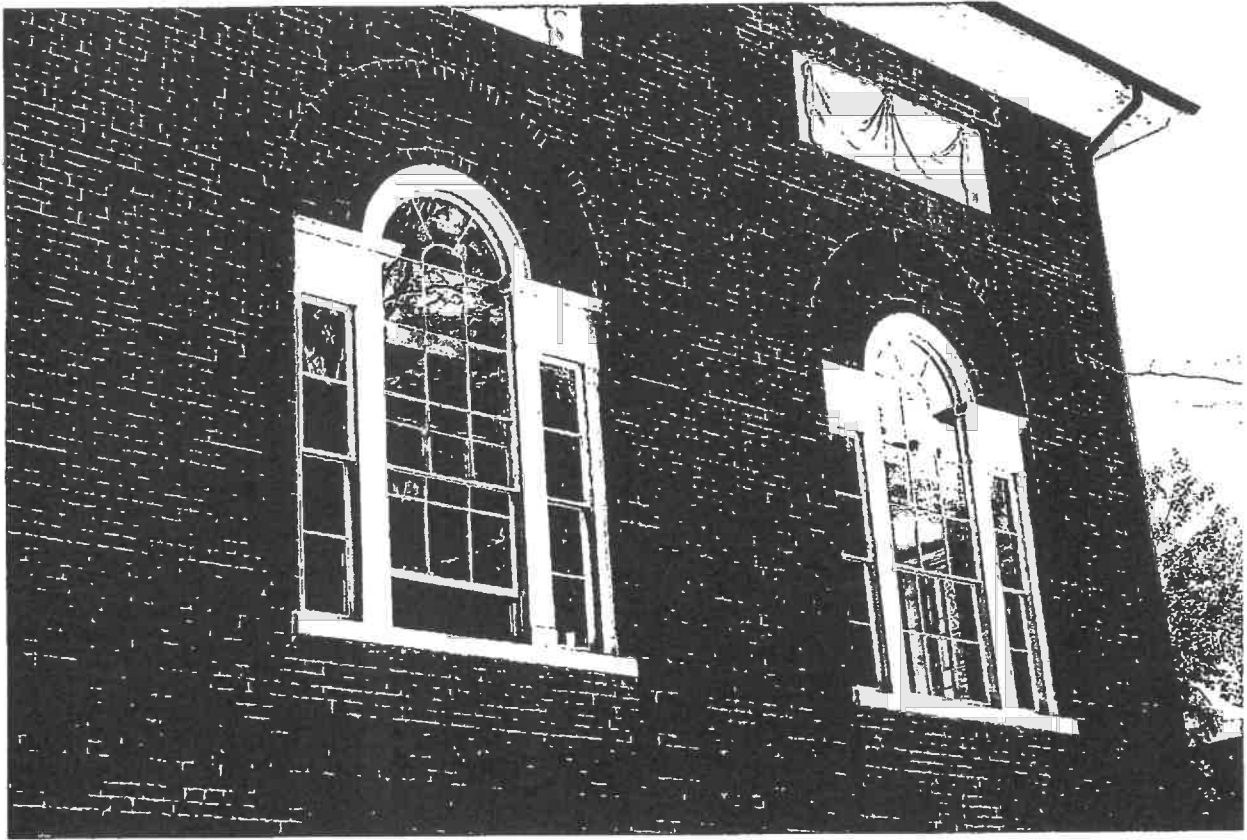
Photo 5: Northwest corner of Chestnut Street façade – Palladian windows and panels with carved swags
