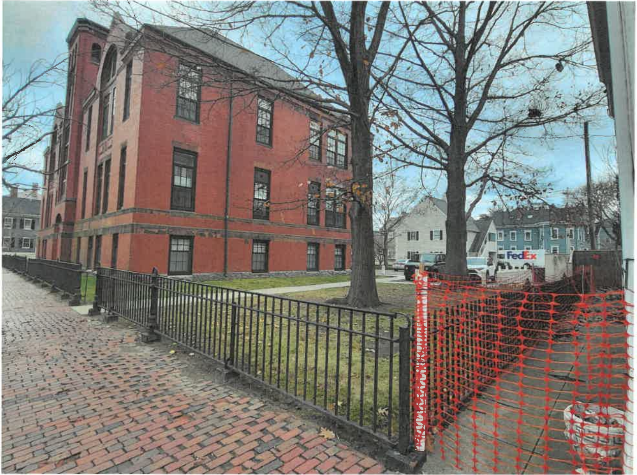
Photo 2- Right side (West elevation) December, 2022
