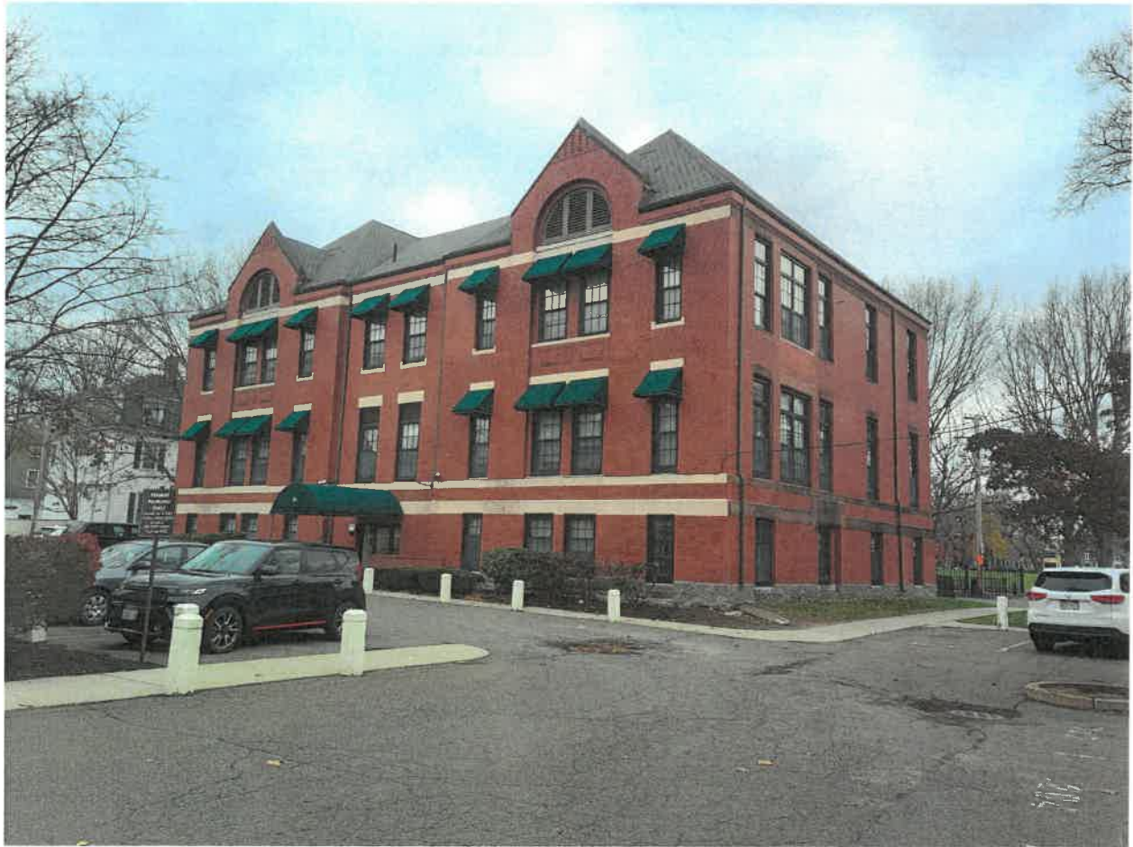
Photo 3- Rear (South elevation) December, 2022
