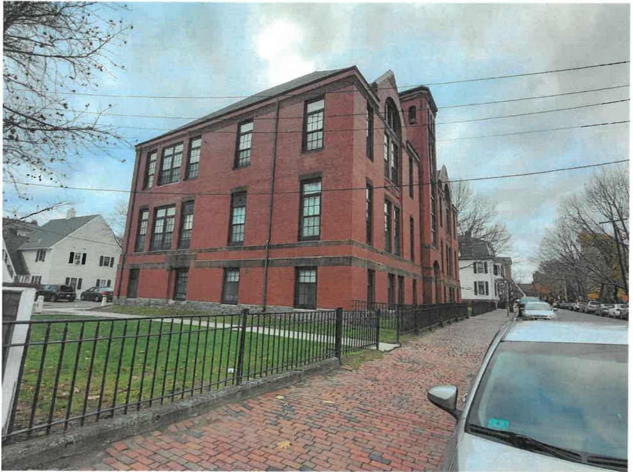
Photo 4- Left side (East elevation) December, 2022
