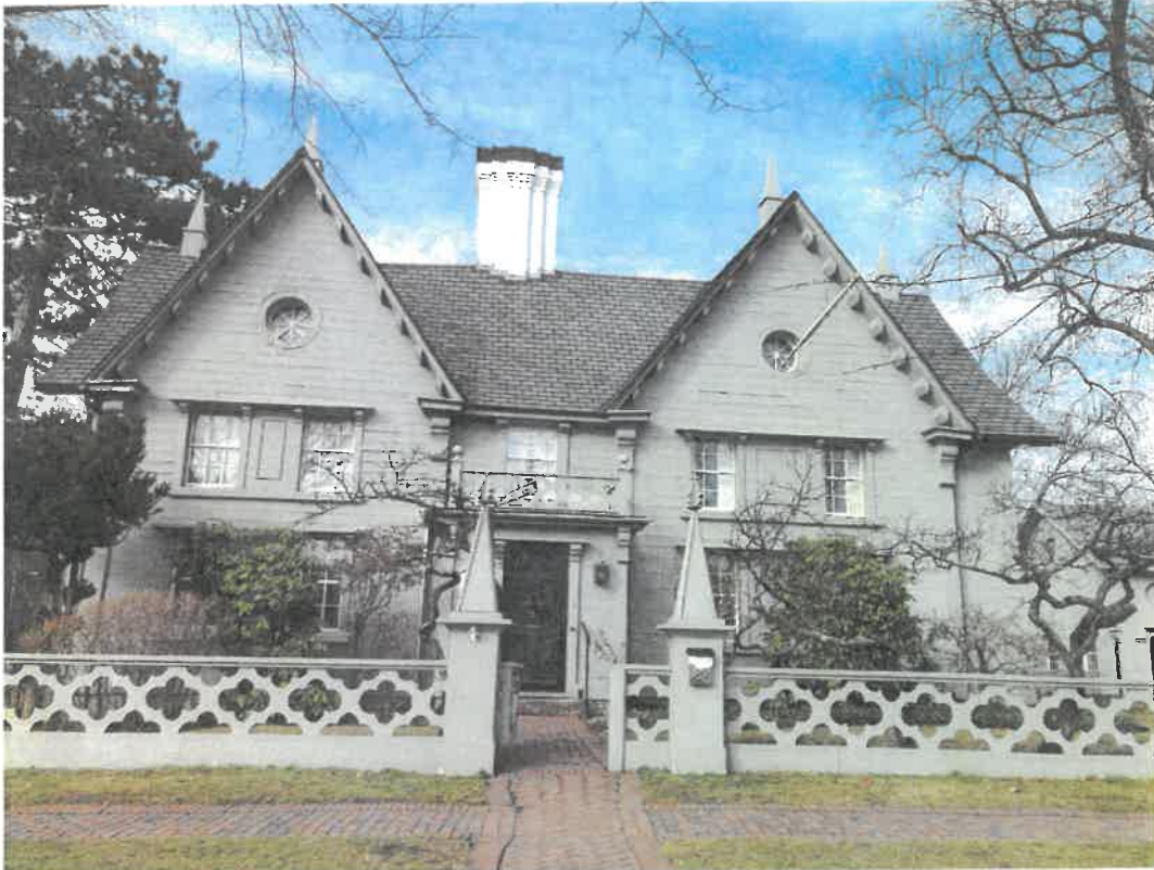
Photo #2: View of front (South) façade, Broad Street
