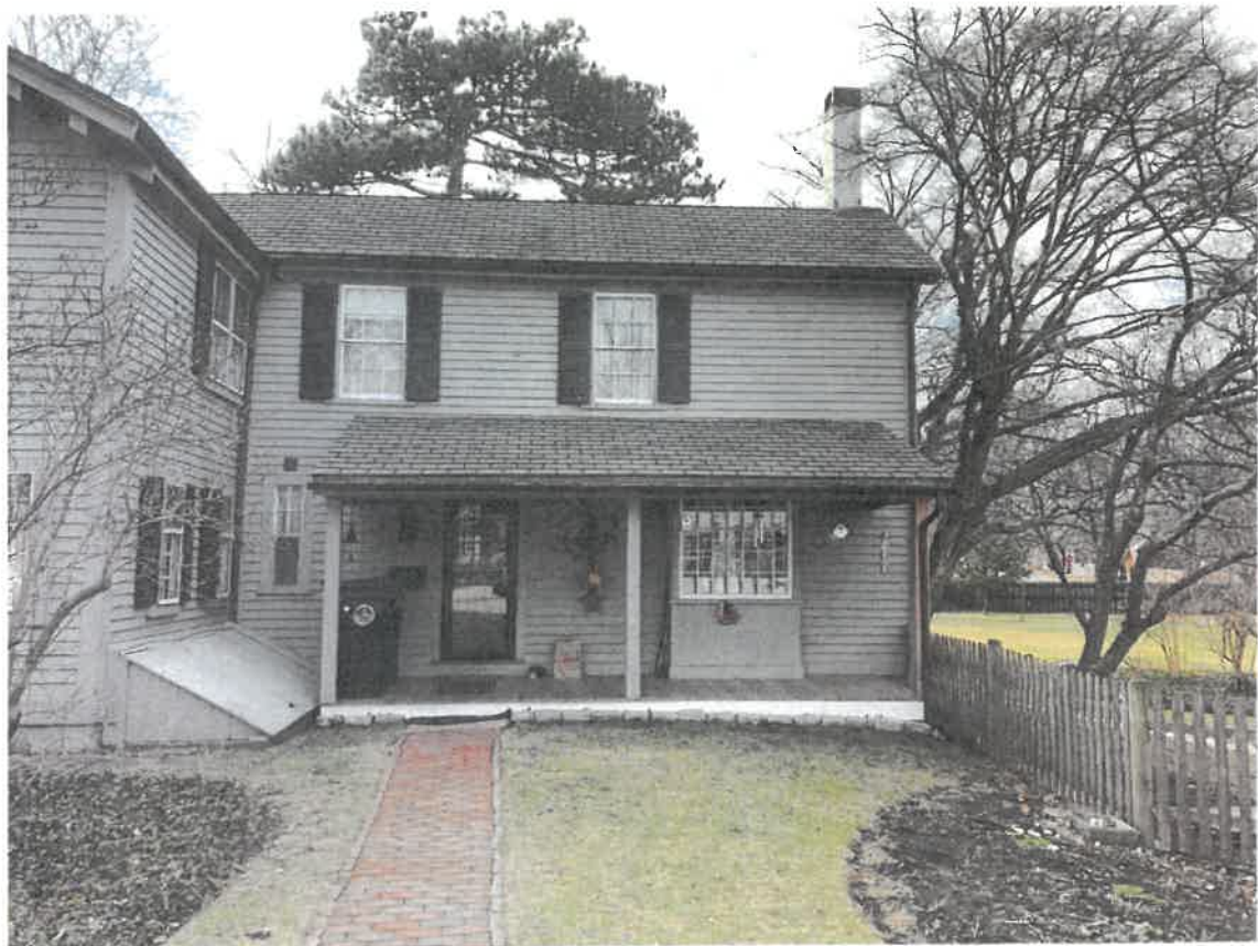
Photo #8: View of rear ell, East elevation
