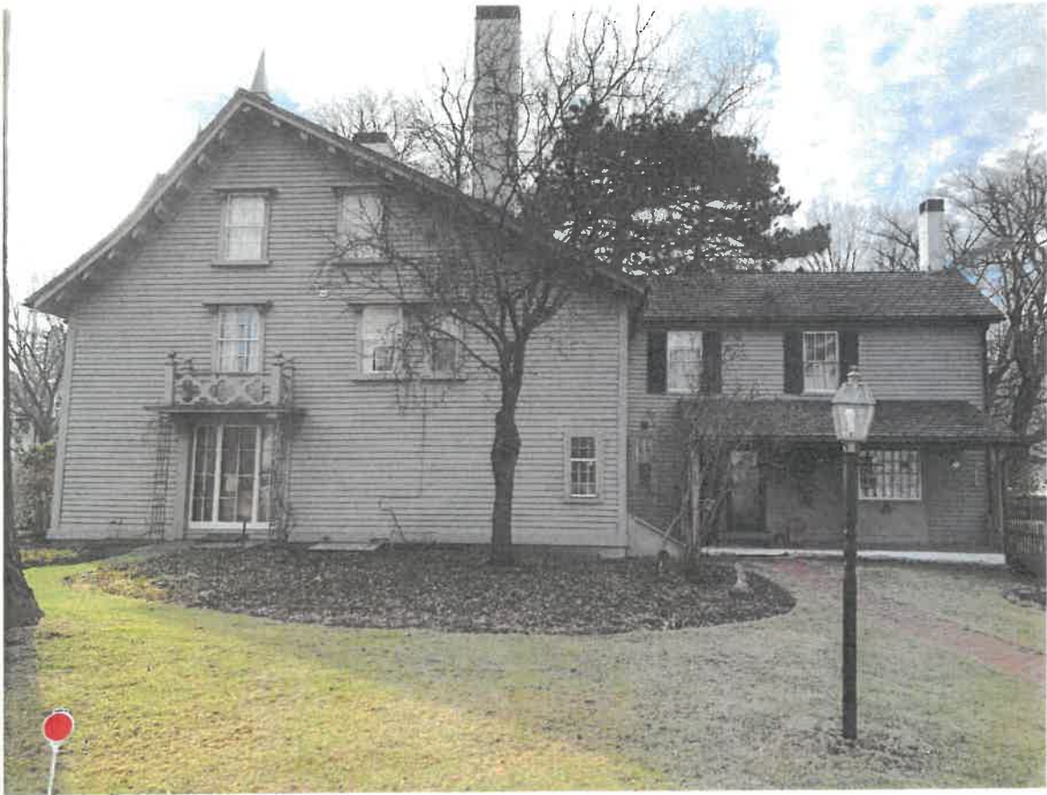
Photo #4: View of East elevation
