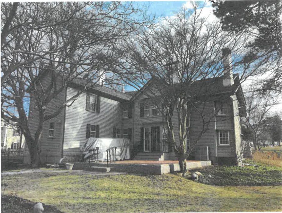
Photo #7: View of North elevation
