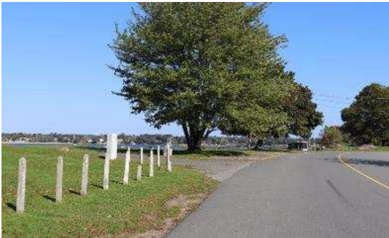
Missing Sidewalk Section
