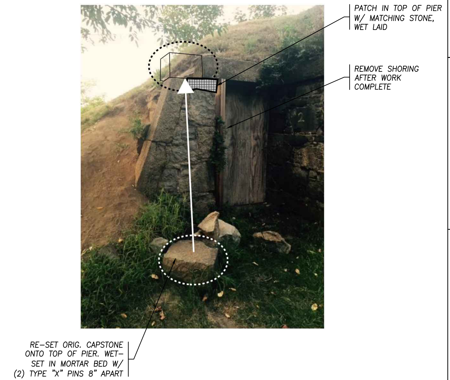
MAGAZINE "C" ENTRANCE REPAIR
