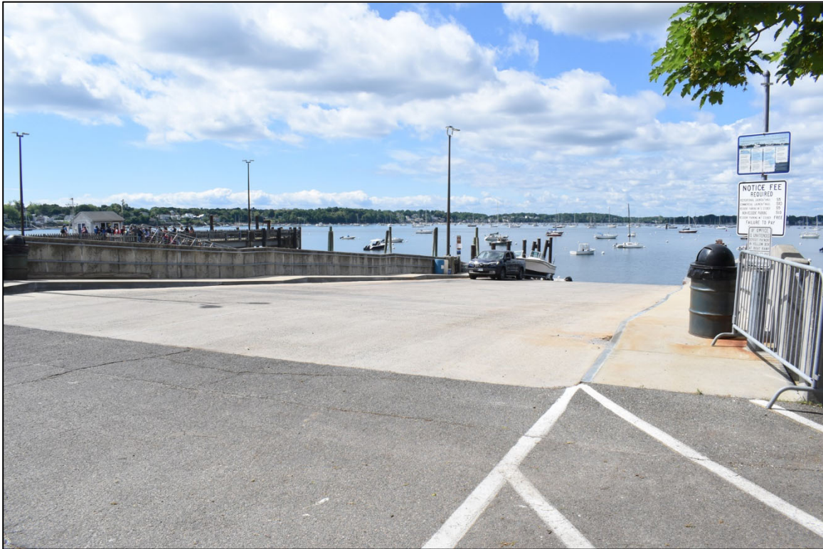
Photo 14. Ramp and Pier, view south from parking lot.
