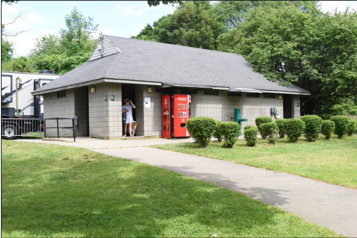
Photo 13. Restrooms/Bathhouse, view north.
