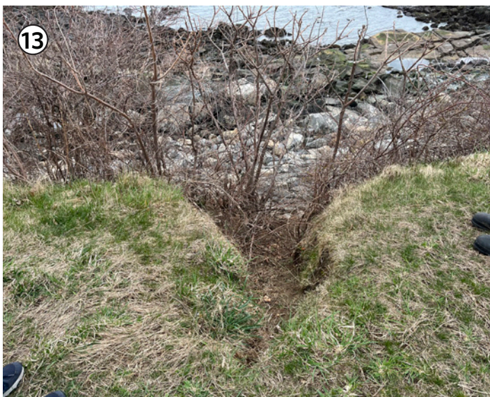
FIGURE 13: ERODED CHANNEL ON THE COASTAL BANK
