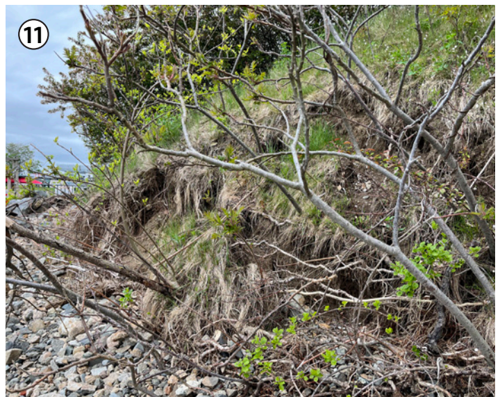
FIGURE 11: SLUMPED SECTION OF COASTAL BANK
