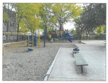
with missing elements on play structures, compacted mulch at the play structures that in some cases sits more than a foot below curbing, and significant erosion on playing fields. As is, Curtis Park is not ADA compliant.
